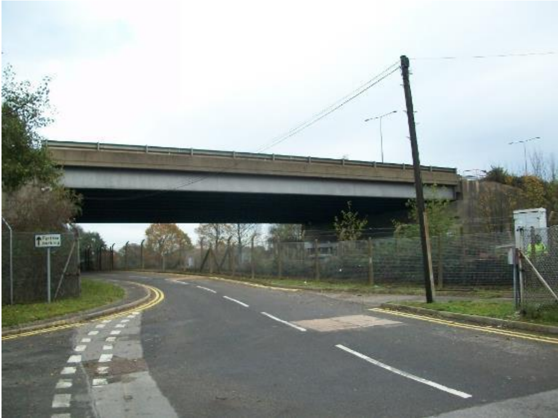
Figure 242423: Existing Airport Way Bridge
