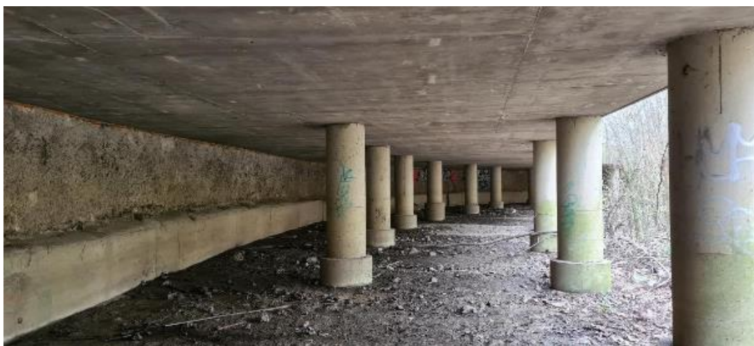
Figure 14 Figure 13 : View from the stilt structure supporting Longbridge SLTL
