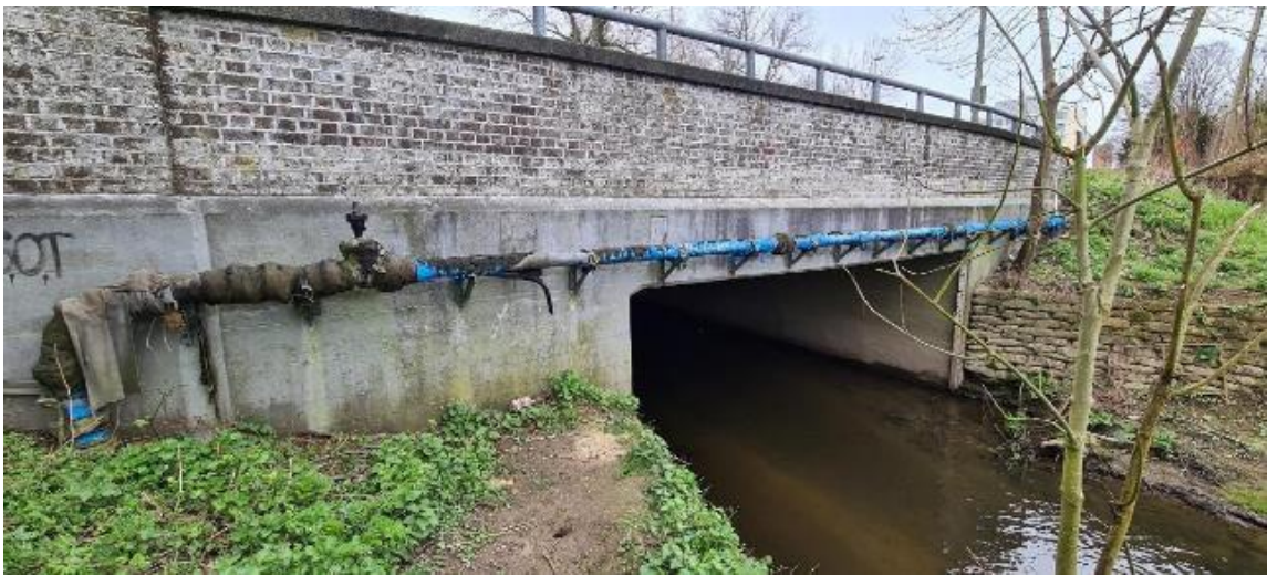
Figure 12 Figure 14 : View of the A23 Brighton Road bridge over the River Mole from the North
